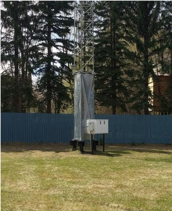
*Photo: Example of similar structure with a climb shield*
