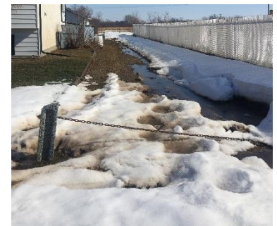
Localized Flooding from Natural Area 2 (March 2019)
