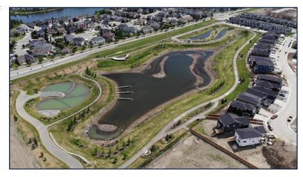
make use of storm infrastructure and allow consistent, high quality reuse potential. Storm Parks specifically approach the challenges of traditional stormwater management and systematically integrate utility, environmental, and amenity value. This alternative approach to stormwater management allows Storm Parks to carefully address site specific constraints and adapt fit-for-purpose objectives on a case-by-case basis.
