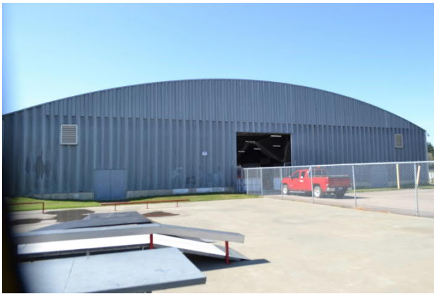
Figure 3-11: Ribbed Corrugated Sheathing Overview
