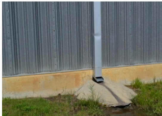
Figure 3-43: Undermined Swale
