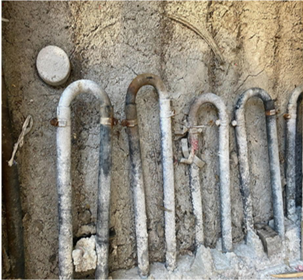
Figure 2-18: Ice Rink Tubes In Slab at North End of Rink
