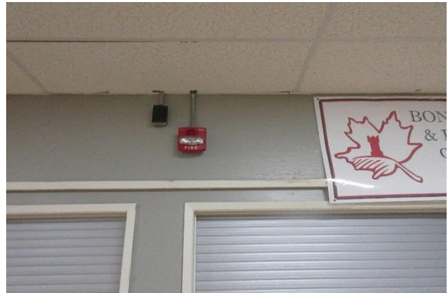
Figure 5-16: Typical Fire Alarm Horn/Strobe
