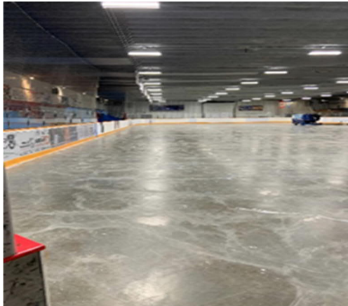
Figure 3-19: Shrinkage Cracking on Ice Arena Slab
