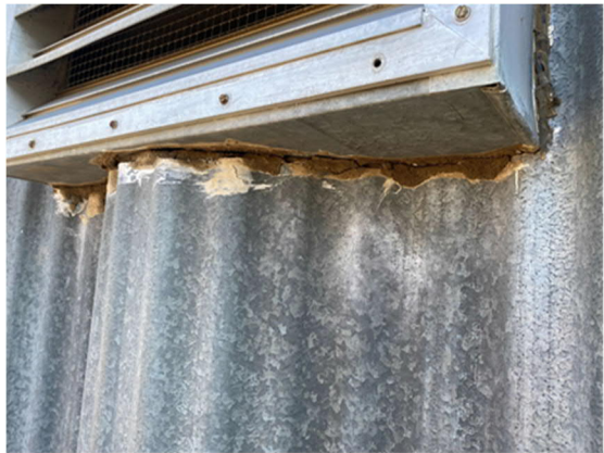
Figure 2-16: Sealant on South Side Air Duct
