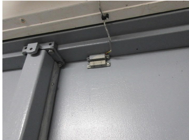
Figure 5-12: Security Door Position Switch
