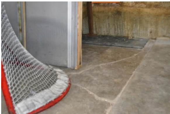
Figure 3-19: Shrinkage Cracking on Ice Arena Slab
