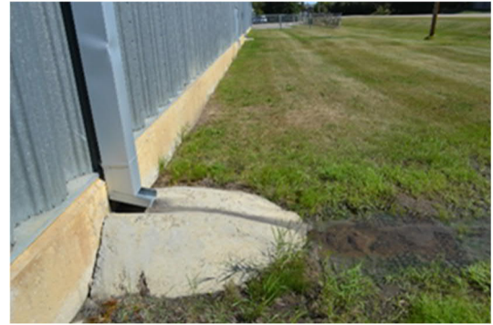
Figure 3-42: Undermined Swale
