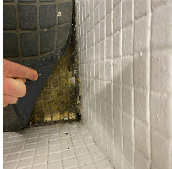
Figure 2-35: Skate Flooring over Existing Showers
