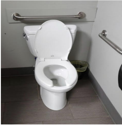
Figure 4-18: Typical 2 nd Floor Water Closet
