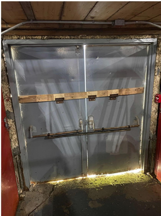
Figure 2-26: Door in East Side beside Bleachers
