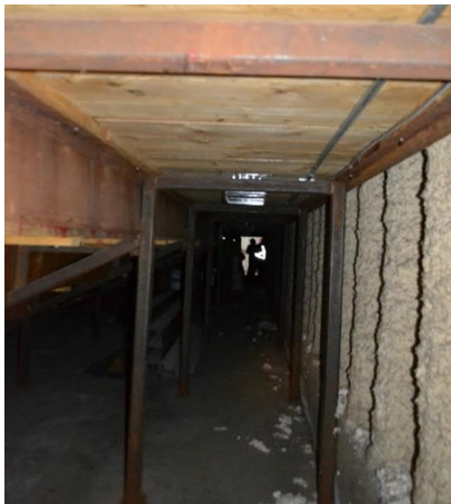
Figure 3-28: Underside of Bleacher Overview
