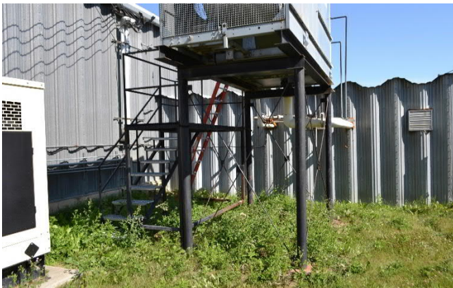
Figure 3-39: Exterior Steel Structure Overview
