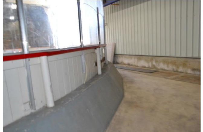
Figure 3-27: Dasher Boards Supports Encased in Concrete
