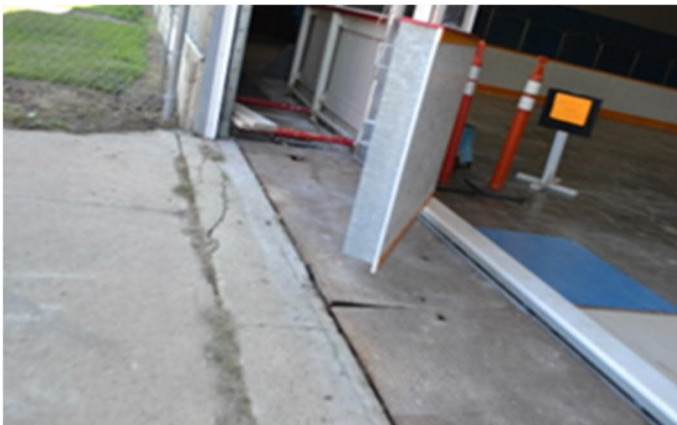
Figure 3-25: Damaged Concrete
