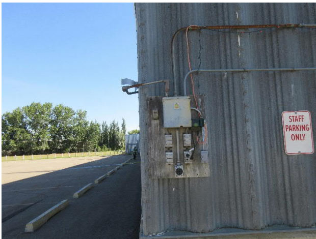
Figure 5-7: Exterior Receptacle
