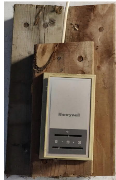
Figure 4-53: Typical Thermostat for Heating Equipment
