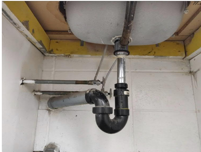
Figure 4-1: Typical Exposed Lavatory Drain
