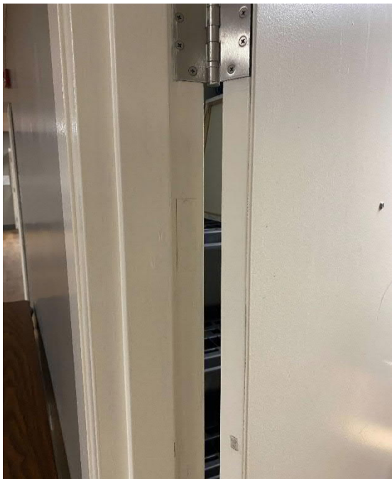
Figure 2-3: Door into Arena - East Side - Rating Covered
