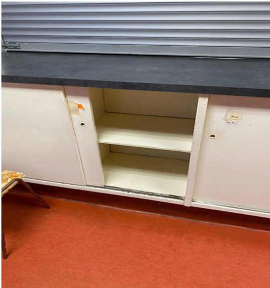
Figure 2-28: Millwork in Concession Area
