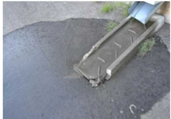
Figure 3-44: Damaged Swale
