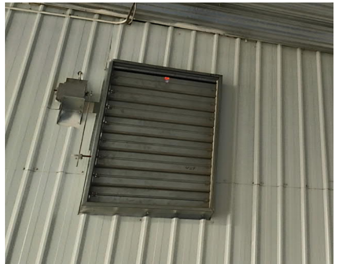
Figure 4-28: Typical Arena Motorized Louvre
