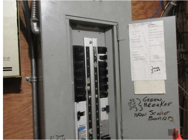
Figure 5-6: Panel B - 200A, 120/208V, 3P, 4W
