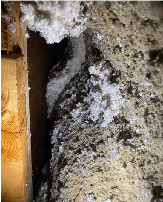
Figure 2-9: Insulation Extending Behind Bleachers
