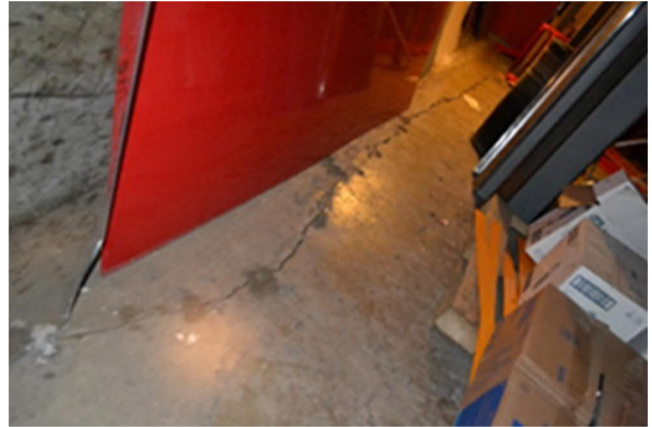
Figure 3-20: Cracked Slab under Bleachers
