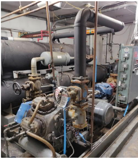
Figure 4-58: Ice Plant Skid
