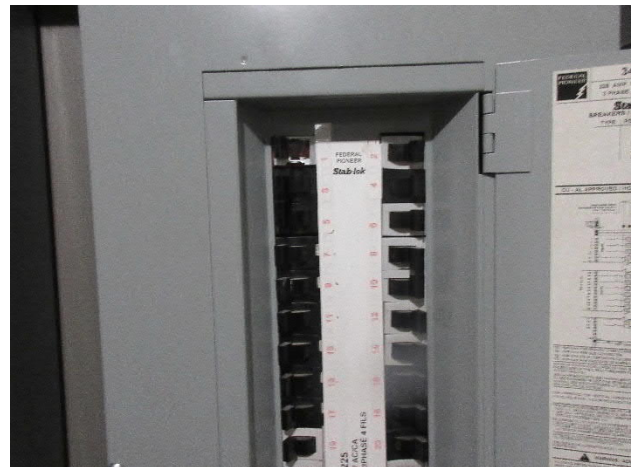
Figure 5-4: Panel EMS - 225A, 120/208V, 3P, 4W
