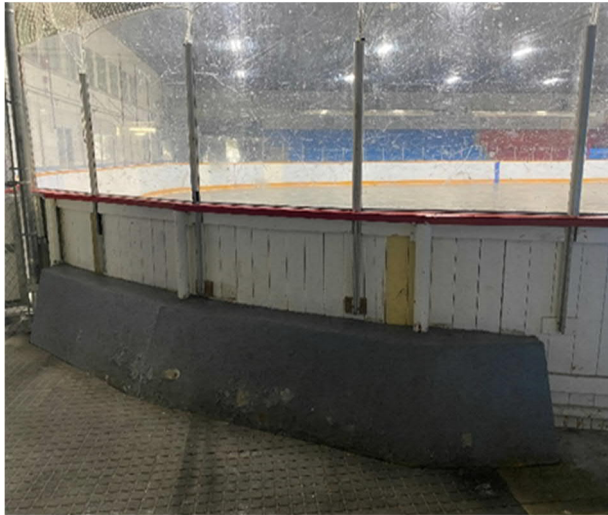
Figure 2-22: Reinforcement at Corners of the Wood Boards
