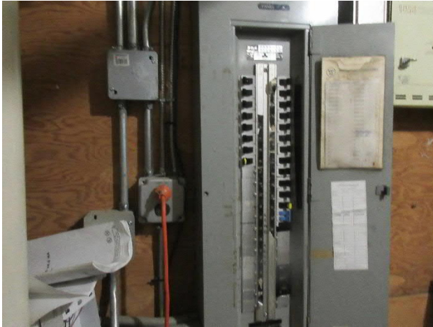
Figure 5-5: Panel A - 200A, 120/208V, 3P, 4W
