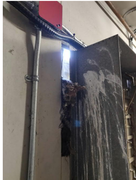
Figure 4-38: Ice Plant Room Louvre Mounting
