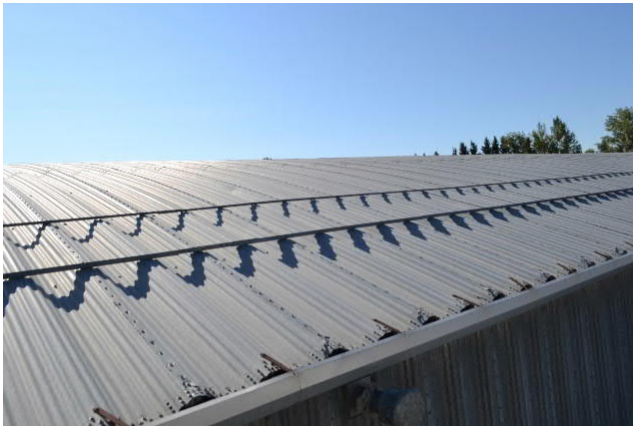
Figure 3-7: Ribbed Corrugated Sheathing Roof Overview
