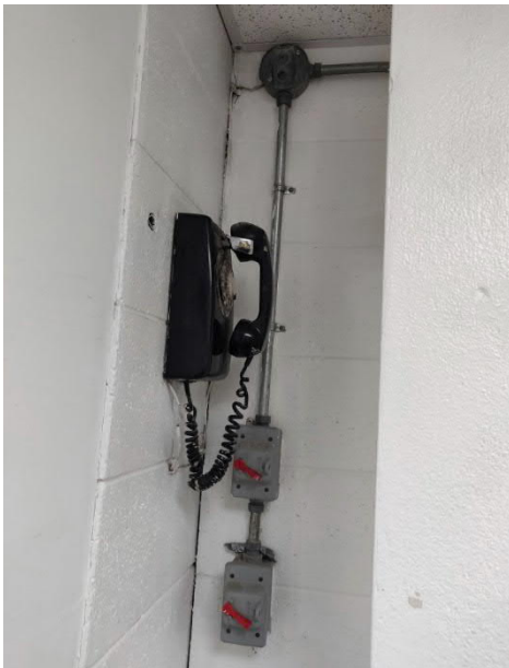
Figure 4-52: Exhaust Fan Control Switches for Arena Exhaust Fans
