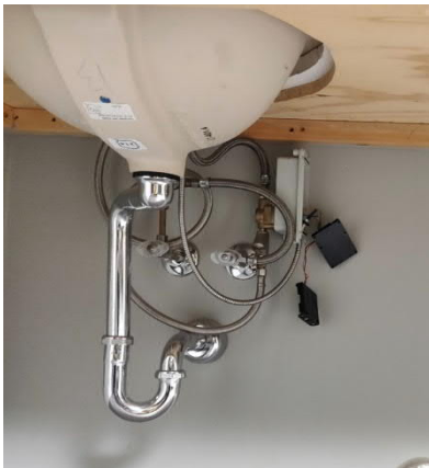
Figure 4-20: 2 nd Floor Lavatory Battery Holster
