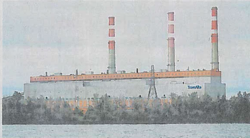
The TransAlta generating plant was the economic engine of Wabamun for decades. LARRY WONG
