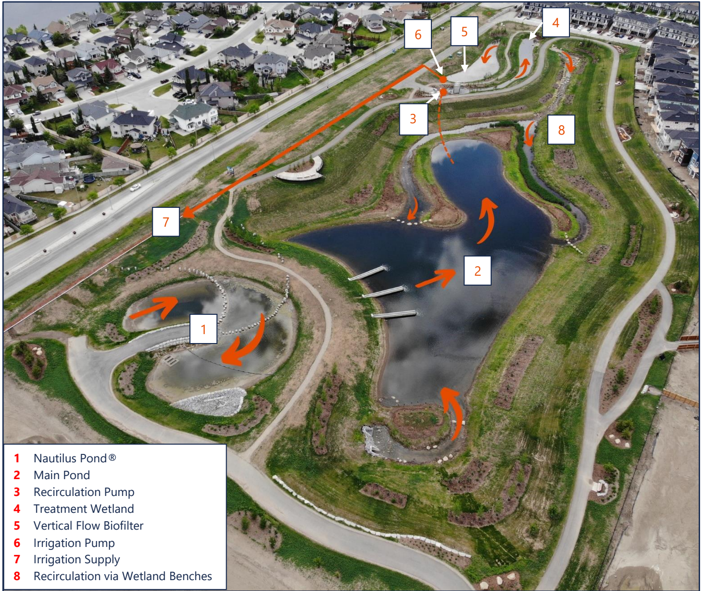
Figure B.1: Pond 2A in operation
